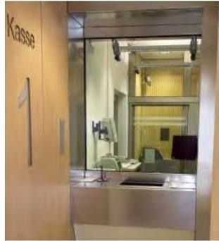
Complete transaction window: fixed field, exchange drawer, intercom.
