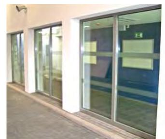
Partition wall within an interlocking door system for the inspection of vehicles (detention facility).
